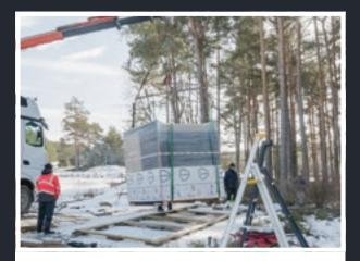
Kirami FinVision<sup>®</sup> Annex modules are delivered to the installation site as whole units, almost fully assembled.
