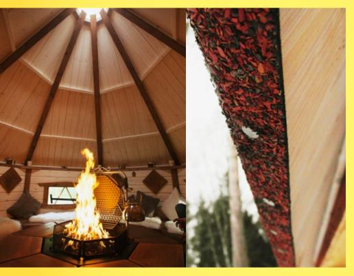
The roof is made with vertical boarding without tongue-and-groove joints to help moisture exit from between the roof boards and felt. We always finish the eaves with drip moulding, which keeps the eaves boarding dry. The wall material is 45-millimetre milled log. The sturdy log helps the building stand strong and will serve you for many years to come.
