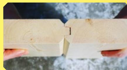
The wall logs consist of one thick joint, which prevents humidity from getting between the logs.
